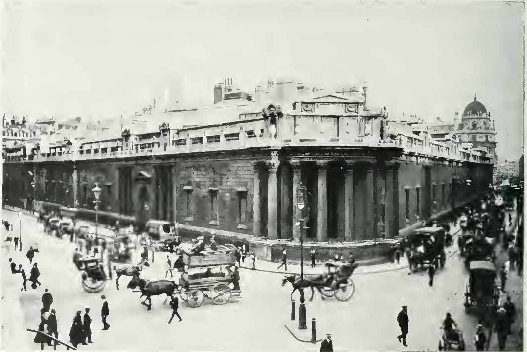
THE MOST BEAUTIFUL ARCHITECTURAL FEATURE OF THE BANK: THE NORTH-WESTERN ANGLE, LOOKING ALONG LOTHBURY (LEFT) AND PRINCES STREET (RIGHT).
